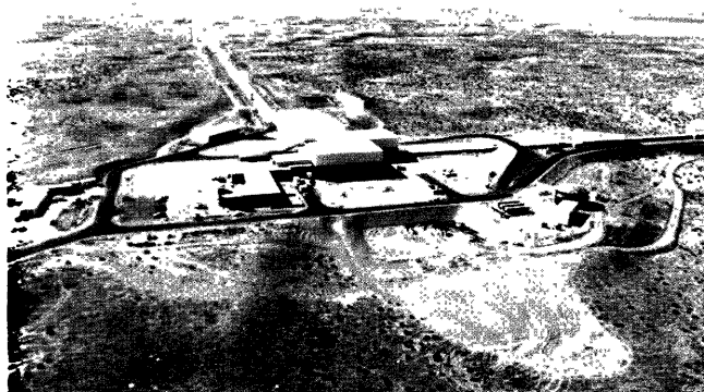
FIGURE 16.5 LIGO gravitational wave detector at Hanford, Washington. LIGO stands for Laser Interferometer Gravitational (Wave) Observatory. The 4-km-long concrete covers of the beam pipes housing the arms of two interferometers can be seen stretching toward the horizon and to the right. The two ends of the interferometer illustrated in Figure 16.3 are at the ends of these pipes. The beam splitter is in the building housing the end station in the foreground. There is a similar facility in Livingston, Louisiana.
