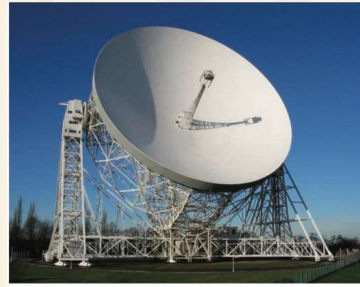
Figure 5.21 The 76-m Lovell Telescope – a prime focus design. Image: Ian Morrison.
