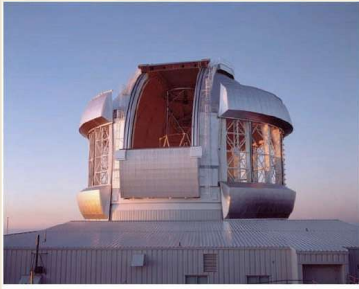
Figure 5.14 The Gemini North telescope. Note the open sides of the dome to allow the telescope to remain in thermal equilibrium with the outside air. Image: Neelon Crawford, Polar Fine Arts, courtesy of Gemini Observatory and National Science Foundation.
